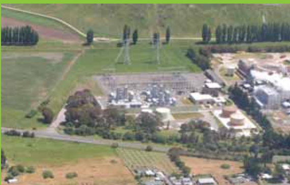
Whirinaki power station. Image courtesy of East Harbour Management Services.
