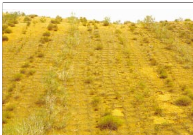
A sand dune stabilized in 1981 with straw checkerboards in Ningxia Province, China
