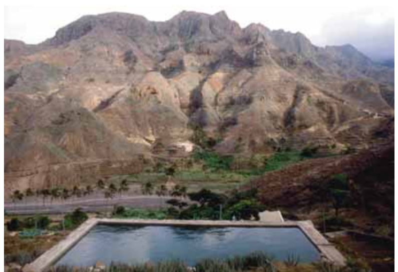
Reservoir for sprinkler irrigation, Ribeira Grande, Cape Verde.
