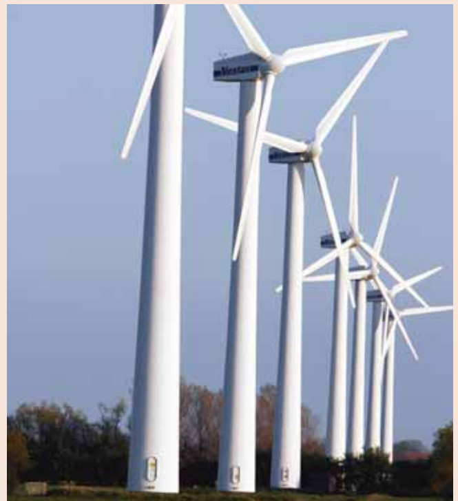
Wind turbine, Germany.
