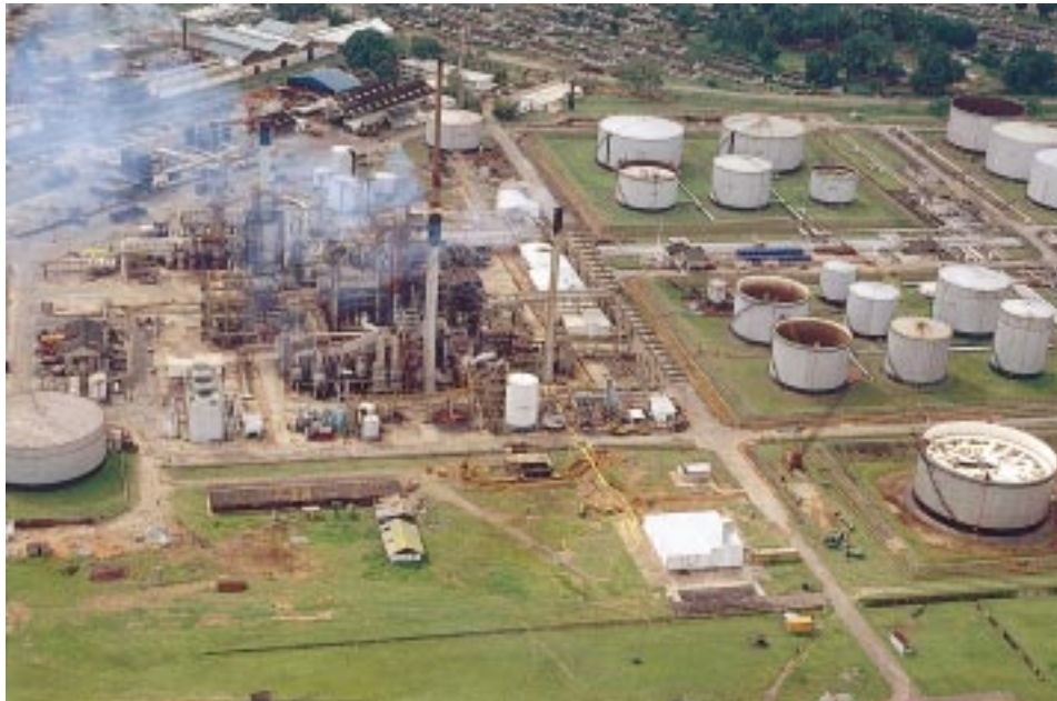
Figure 49 : Oil refinery at Mombasa
