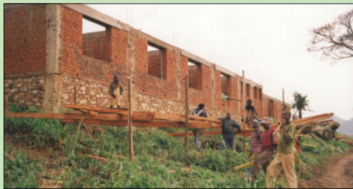
The Tayna Center for Conservation Biology under construction
