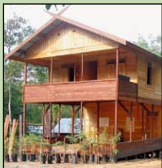
Training centre/guard post in Belantikan
