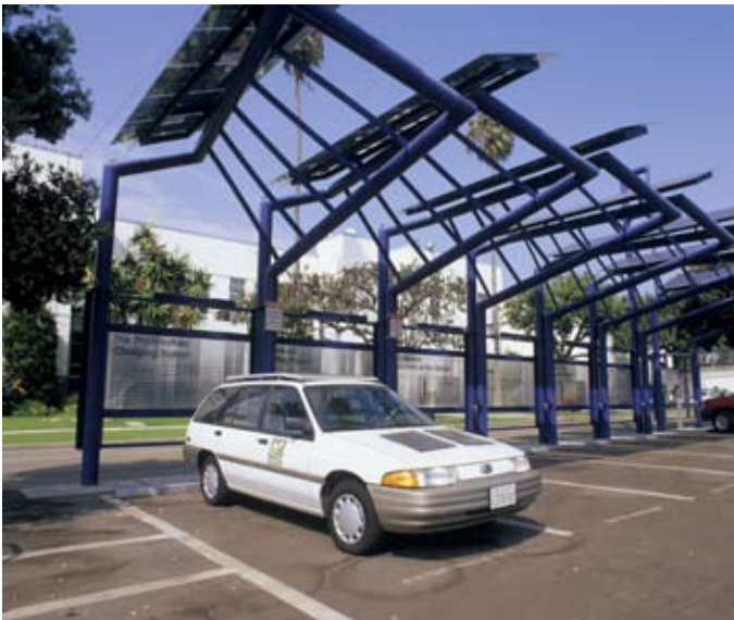
© Martin Bond / Still Pictures Electric car charging station powered by solar energy. City Hall, Santa Monica, California, USA.
