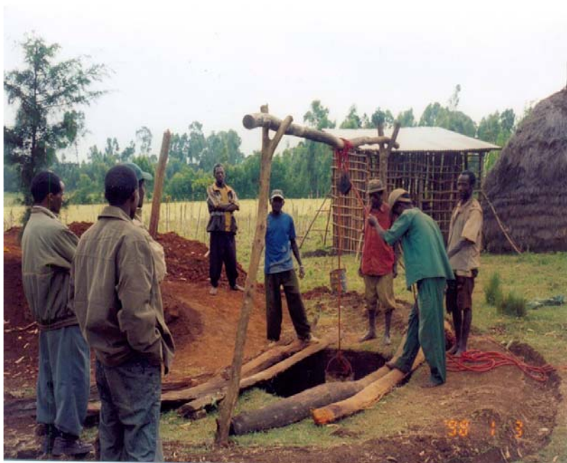
Illustration 21: Construction de pompe manuelle
