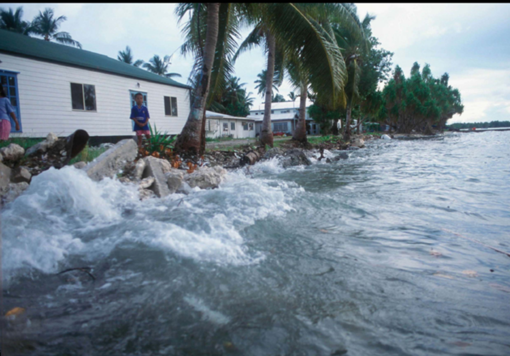
Photograph by Erika Perdomo. Taken from the island of Tuvalu and being approximately 100m from the shore. The building belongs to the Tuvalu Government Ministry of Health. June 2007.
