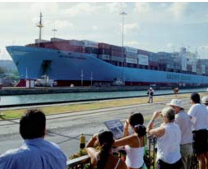
A container ship moves through the Miraflores locks of the Panama Canal which are supplied with fresh water from upland reservoirs to float the ships.
